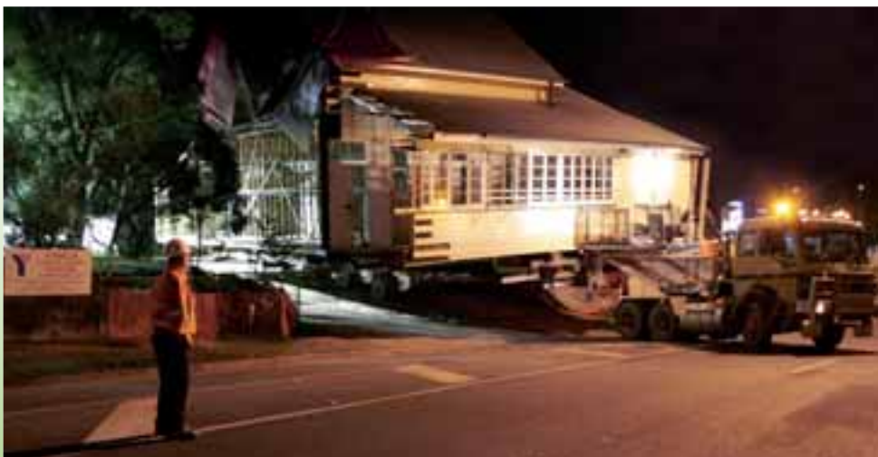
Relocating the School of Arts Building during the early hours of the morning, 15 November 2008
