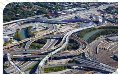
Top: Airport Link cut-and-cover tunnel portal
