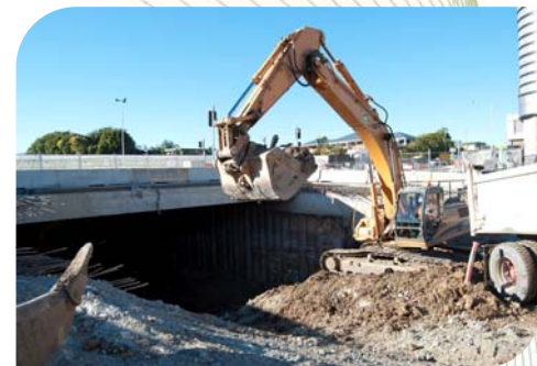
Top: Completion of jack box operation
