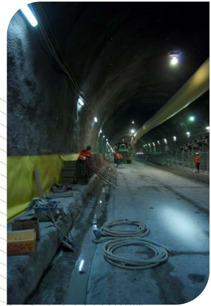
Top: Eastbound tunnel footers
