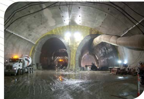
Top: Installation of steelwork for TBM burial chamber
