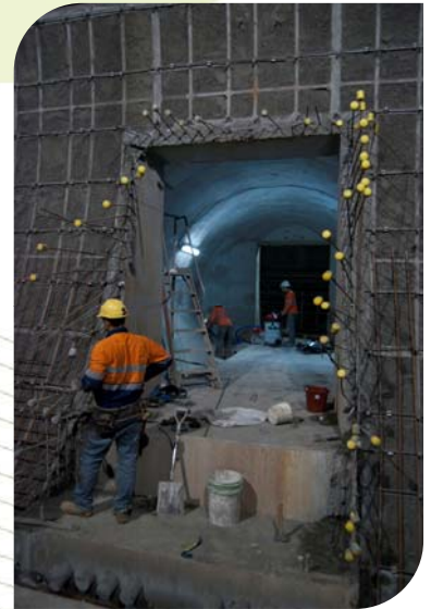
Above: Mechanical and electrical fit-out of TBM tunnel cross passage
