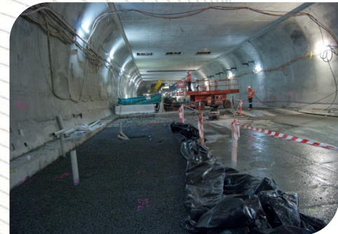
Top: Demobilisation of the acoustic shed
