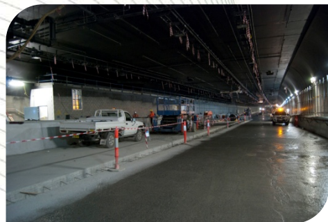
Top: Signage installation on Airport Link bridge connections
