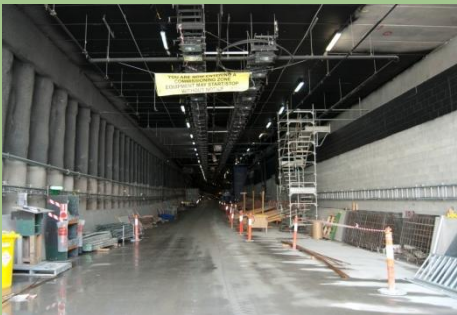
Northern Busway Tunnel – Lutwyche to Kedron
