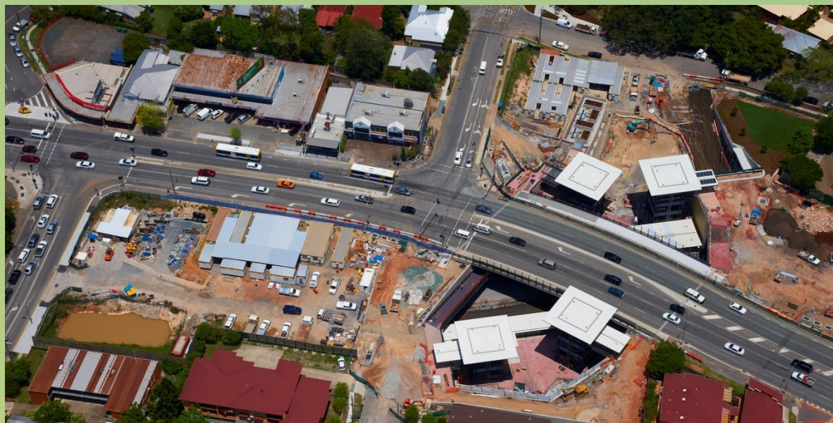
Aerial – Lutwyche Busway Station Site December 2011
