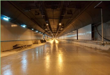
Airport Link Tunnel
