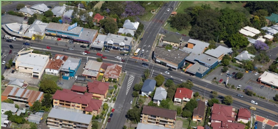
Aerial – Lutwyche Busway Station Site October 2008
