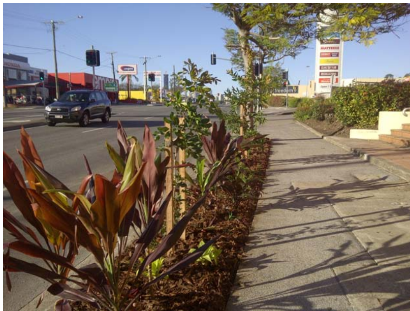
Lutwyche Road footpath upgrade
