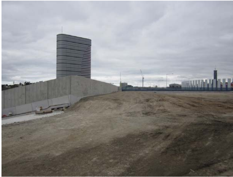
Backfill on top of cut and cover structure
