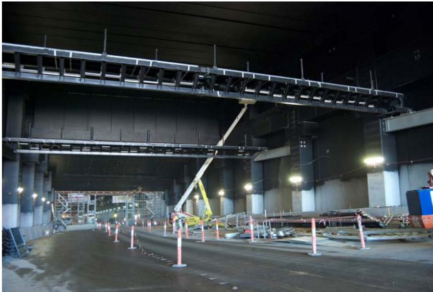
Mechanical and electrical fit out - tolling gantries
