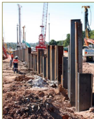
Sheet piling (above) and bored piling (right)
