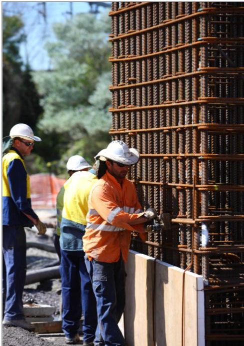
Diaphragm walling: installation of steel reinforcement cage
