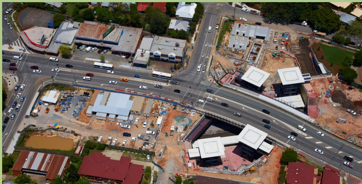
Aerial – Lutwyche Busway Station Site December 2011
