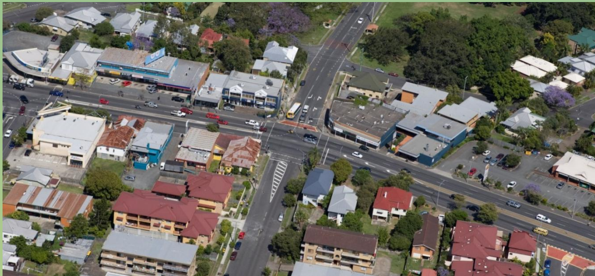
Aerial – Lutwyche Busway Station Site October 2008
