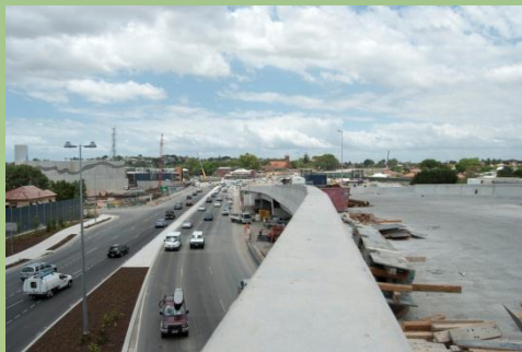
Gympie Road Flyover
