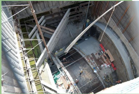
Eastbound Tunnel at Kedron Central Site
