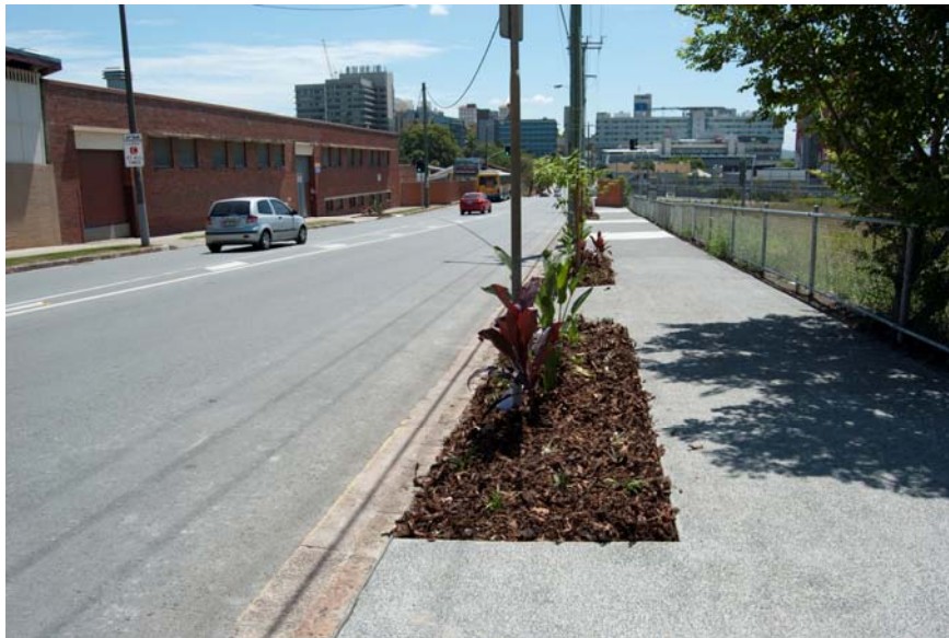
O'Connell Terrace Footpath Reinstatement
