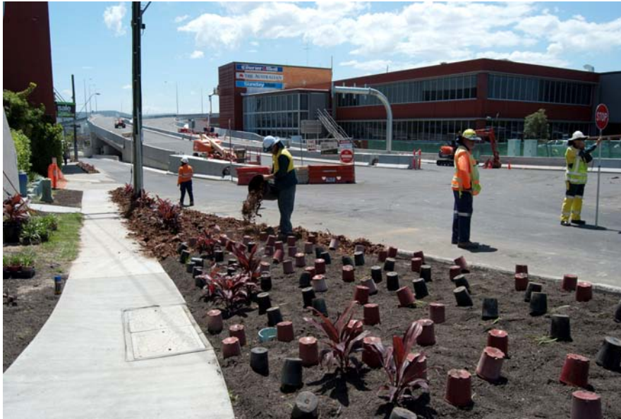
Airport Link on/off-ramp to ICB and Campbell Street
