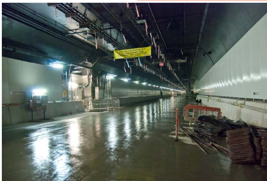
Mechanical &amp; electrical fit out and commissioning
