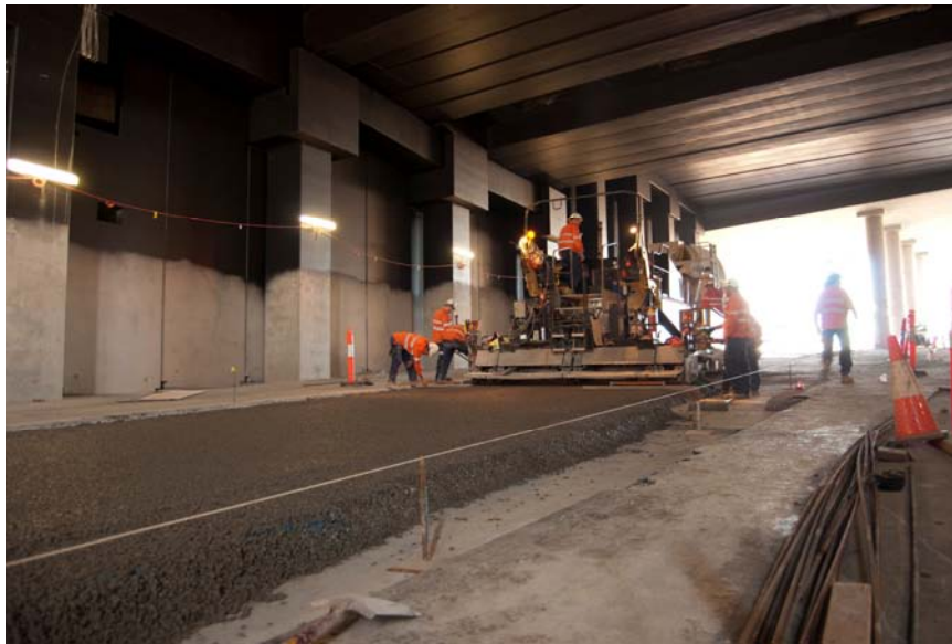
Installation of concrete pavements tunnel portal
