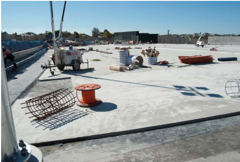
Cut and cover tunnel roof preparation for hill-top park backfill
