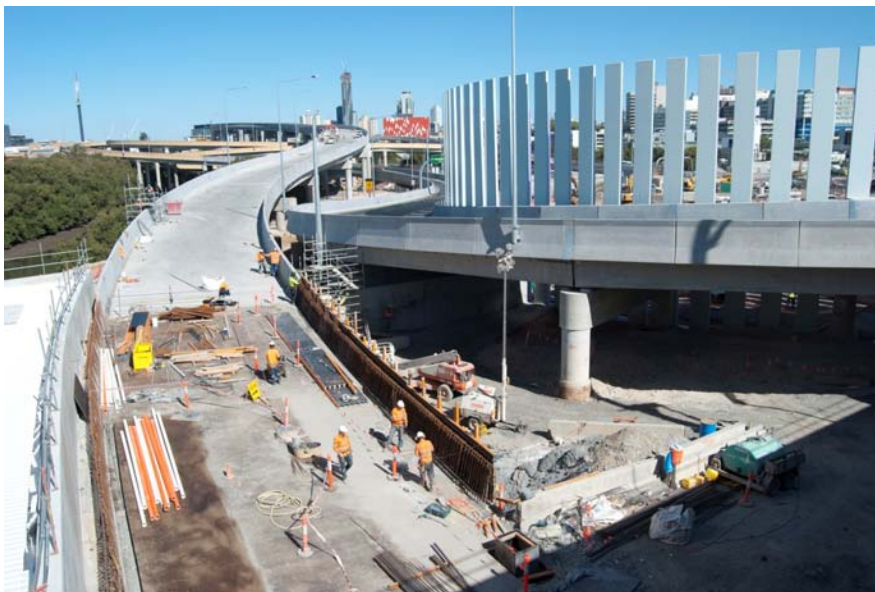
Southbound Airport Link off-ramp to ICB and Campbell Street
