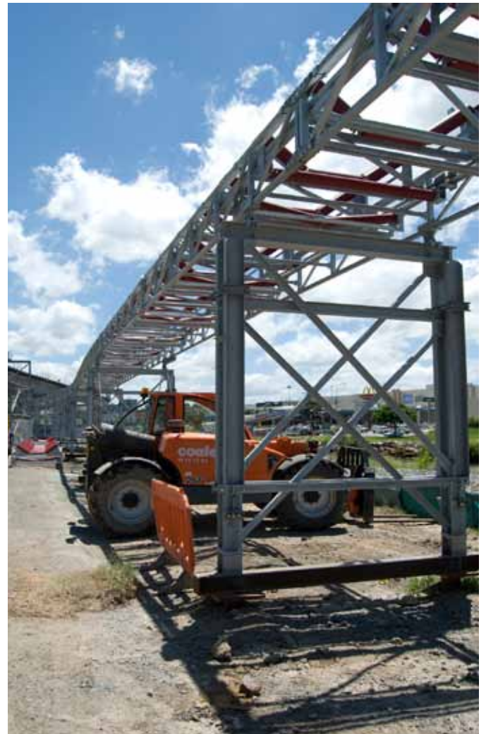
Construction of TBM spoil conveyor
