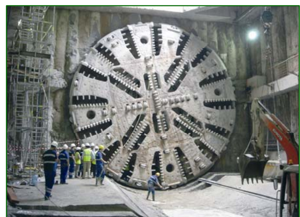
Two TBMs will be launched from Toombul
