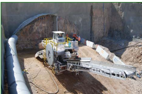
Eleven roadheaders will be used on the project
