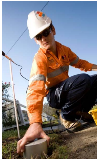
Installation of vibration monitor
